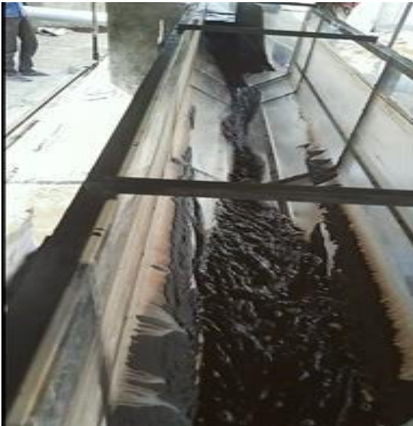
Photograph 3. Flushing in progress after closure of inlet gate
