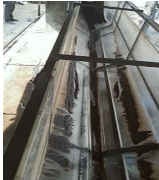
Photograph 4. After complete flushing is achieved
