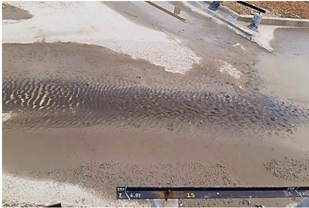
Photograph 5. Before Diversion (Existing Situation)
